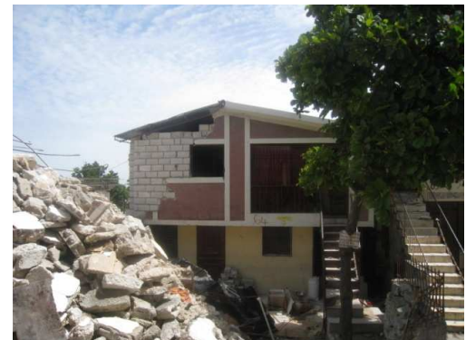
Rubble next to a house being repaired.
