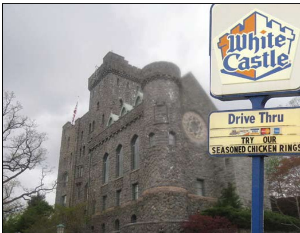
Adaptive re-use may take a medieval structure like The Castle on the Hudson in Tarrytown (above) and transform it into a castle of a very different kind, a White Castle.
